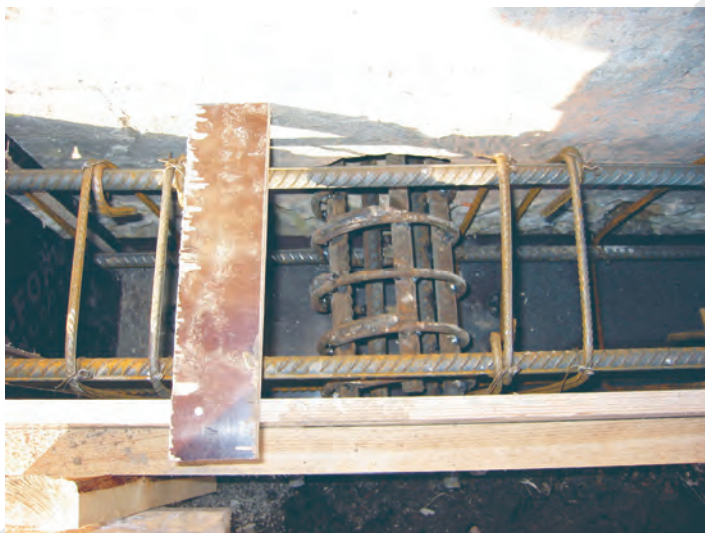
Reinforcement for the concrete waling.
