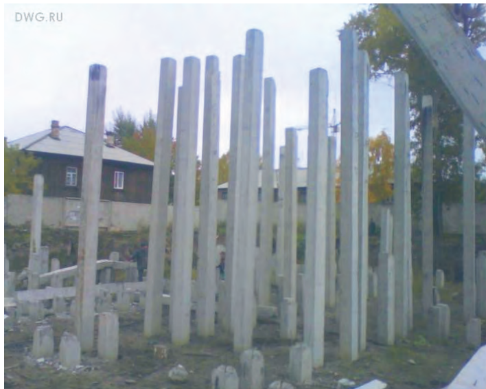
Pile forest instead of pile field.
