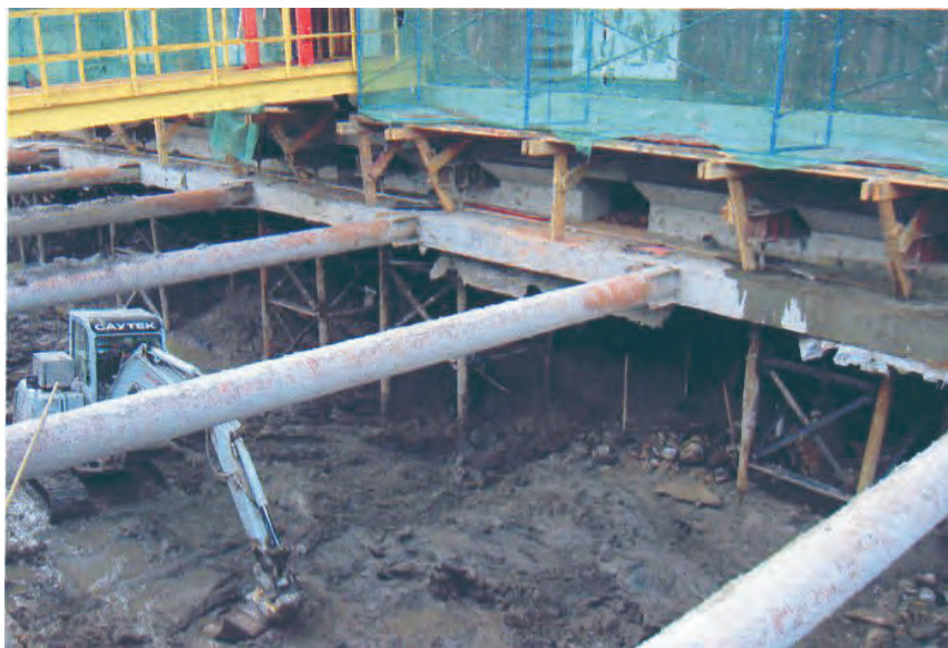
Struts constructed of steel pipes have been placed between the top slab and the sheet pile wall. Excavation under and around the theatre is underway.
