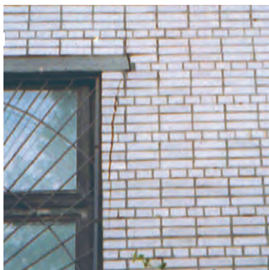
The characteristic outlook of settlement-related cracks for buildings with reinforced concrete crosspieces: left – according to numerical analyses; right – on the building adjoining the accident site (Dvinskaya 8, Building 2).
