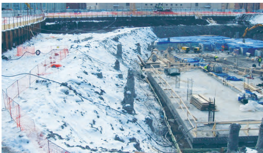
Excavation with slopes.
