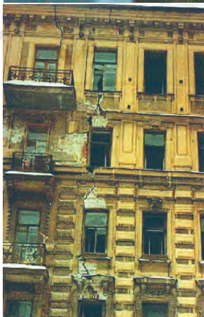
Examples of destruction caused to historic buildings during construction of underground volumes for “Nevsky Palace Hotel” on Nevsky Avenue (top left and right), and an apartment house on Michurinskaya Street.
