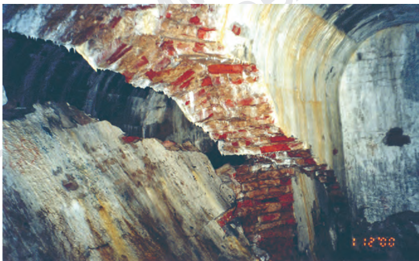
Cross-section walls of the retaining structure, forming a terrace in front of the palace, as witnessed by condition surveyors.
