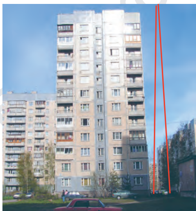
Consequences of trying to save on pile lengths: a tilting house, cracking panels, settlements of about 0,5 m!
