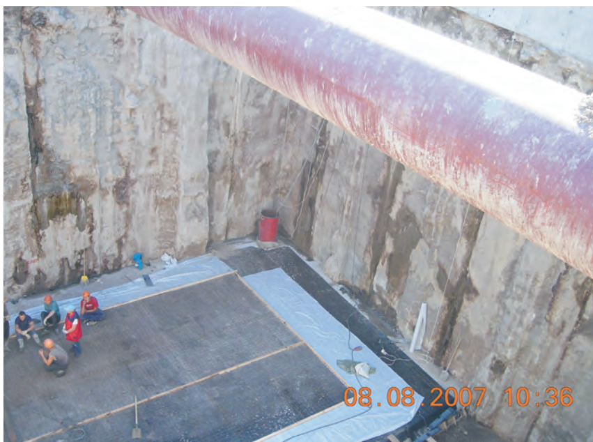
The first ever successful trial of diaphragm wall protected excavation in St. Petersburg on the Orloff Tunnel site.
