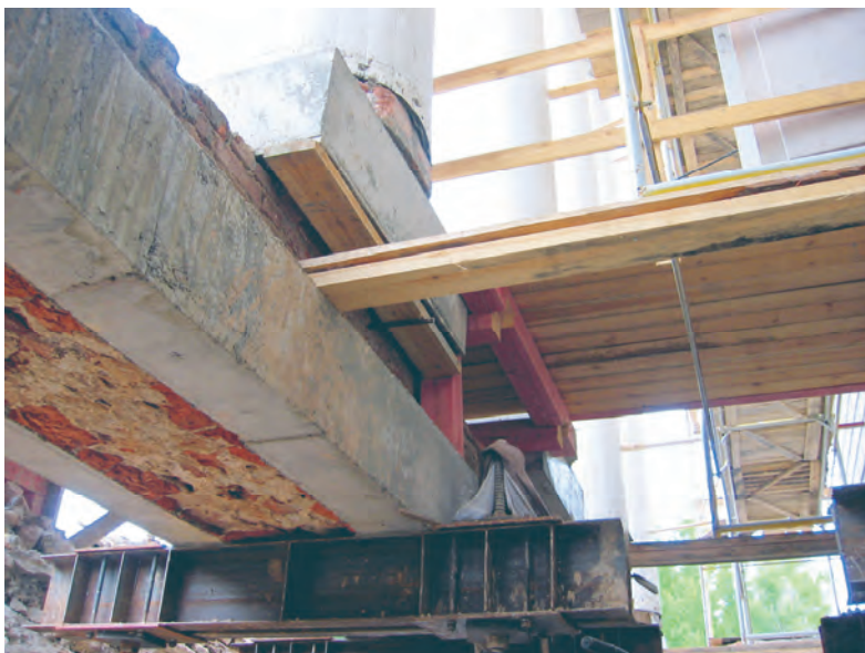
All loading is transferred to piles. The old foundations are removed (the photo also illustrates the point of view of a geotechnical engineer on architecture).
