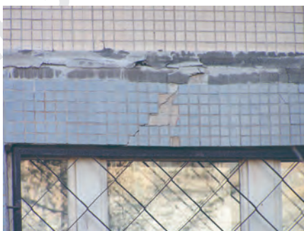
Consequences of trying to save on pile lengths: a tilting house, cracking panels, settlements of about 0,5 m!
