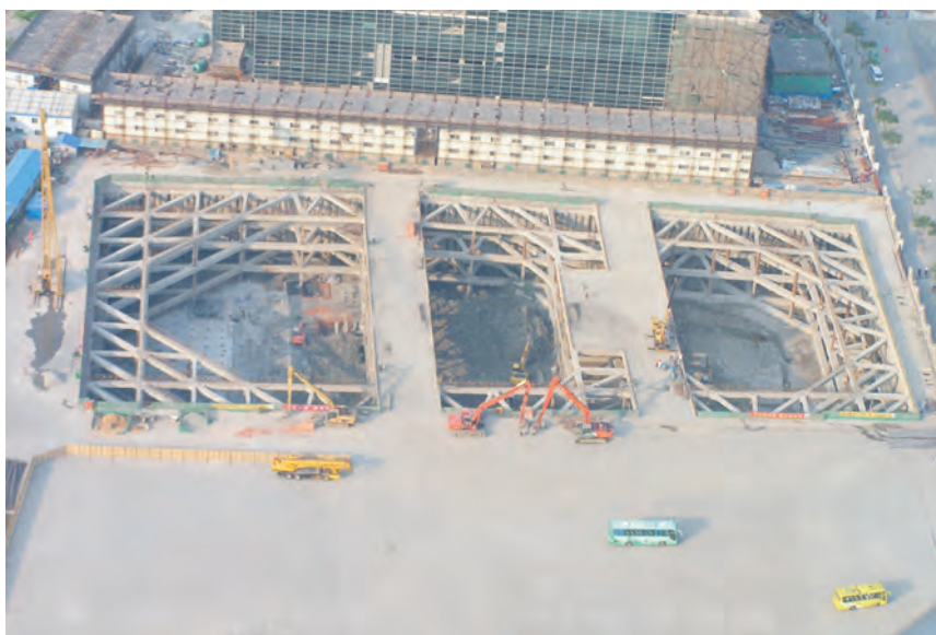
Temporary reinforced concrete props on an underground construction site in Shanghai.
