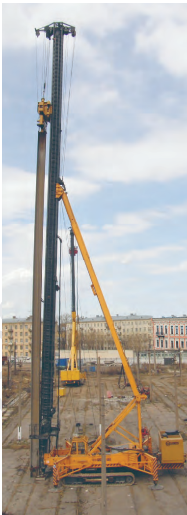
Vibratory driving of record length sheet piles.
