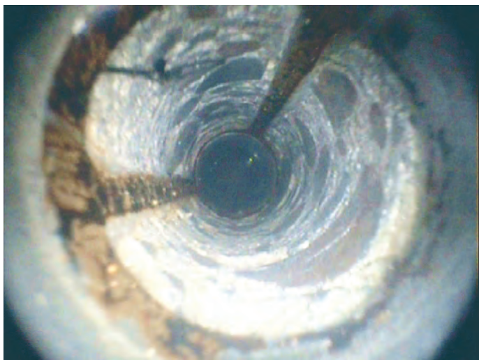
A metallic structure in the foundation body at the depth of 0,6 m (a miniature camera photography inside a borehole).
