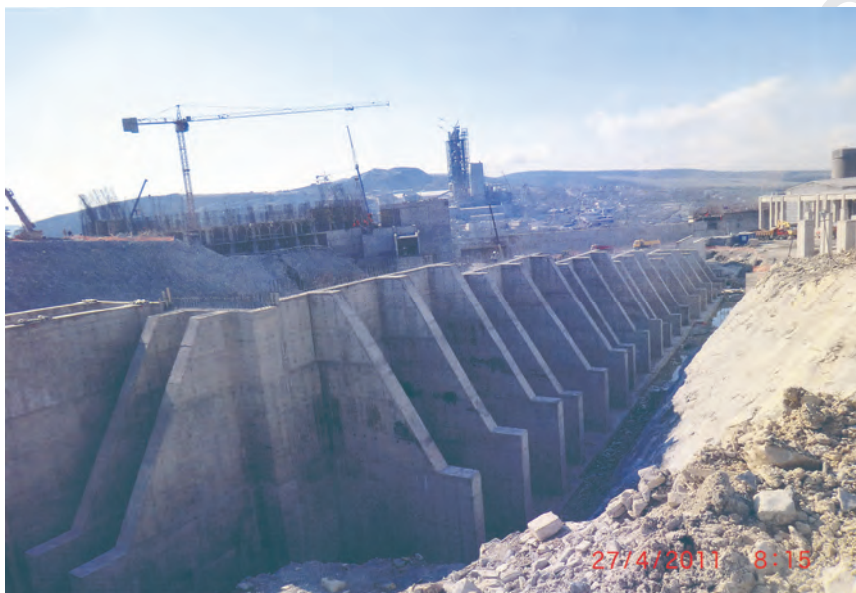
A 20 m tall retaining wall; a terrace of cement production plant in Novorossiysk.
