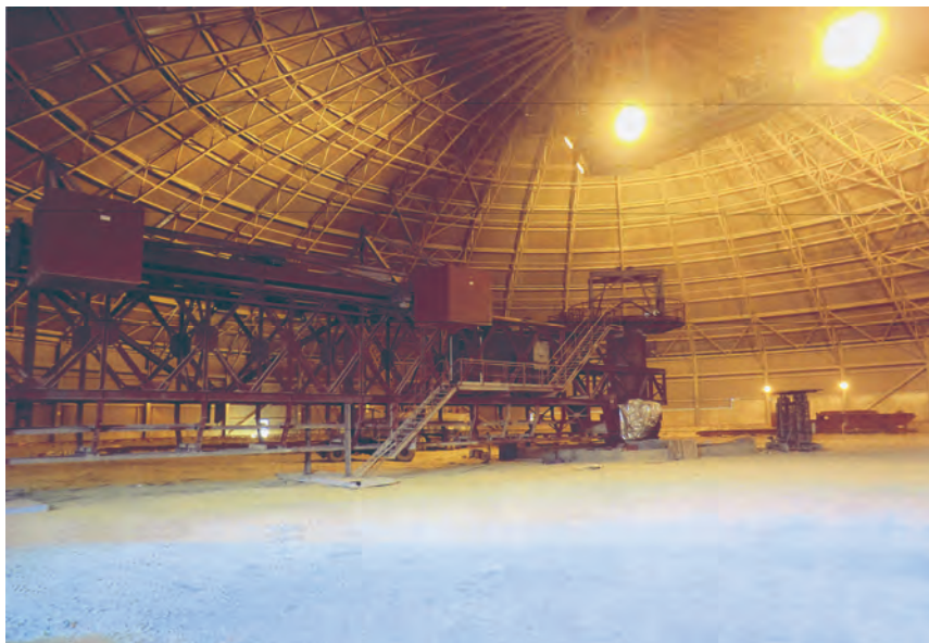
Clinker storage facility: the inside view.
