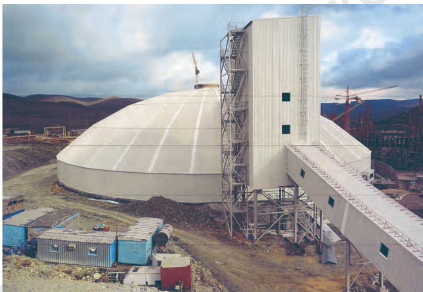
Clinker storage facility: a dome 100 m in diameter.
