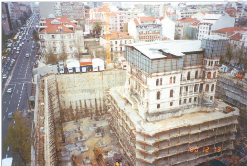
A. Pinto: construction of an underground volume around a historic building in Portugal.
