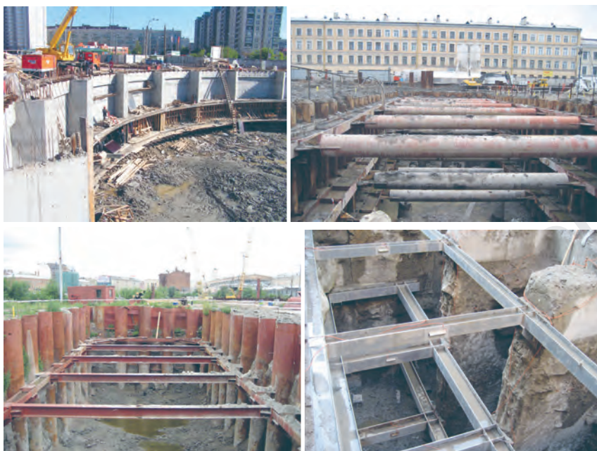
Fully instrumented deep excavation test pits in St. Petersburg with detailed monitoring of soil behaviour.
