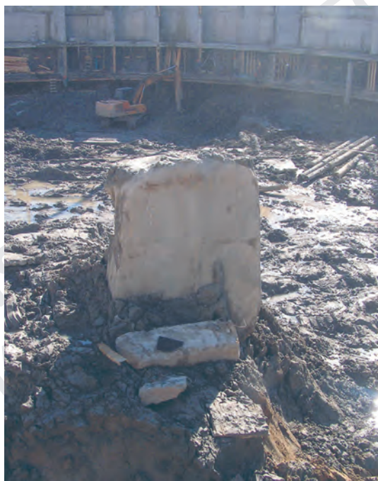
First trial to construct diaphragm wall according to modern technology (Franki, Geoizol, Komendantskaya Square).
