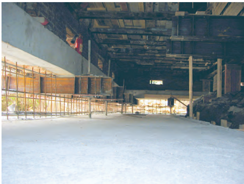
Placement of the top slab.
