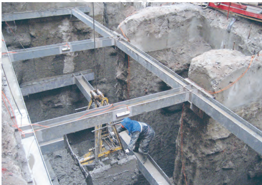
Zoologichesky Lane. First trial of diaphragm wall construction in adjacency to existing buildings (the experiment was carried out on the buildings subject to demolition).
