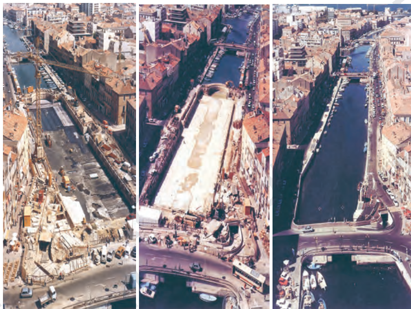
Soletanche-Bachy: construction of a two-storeyed parking lot below the river bed in a historic city in France; from left to right: construction of a waterproofing for the parking floor (the river water is temporarily running through a pipe); stacking of protective slabs – the artificial river bed; completion of construction, of which one is reminded only by the parking entry gates.
