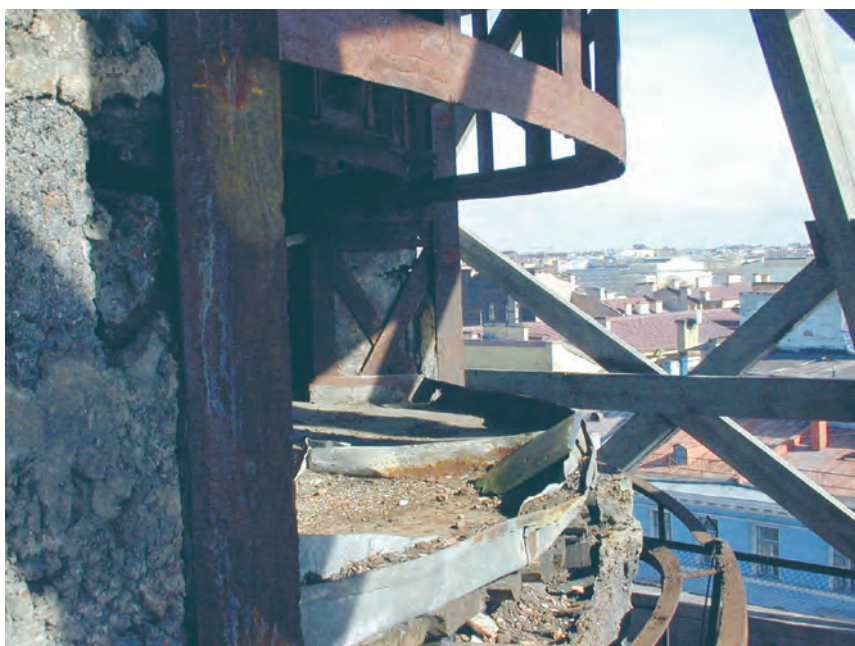
Steelwork inside the masonry of the "Book House".
