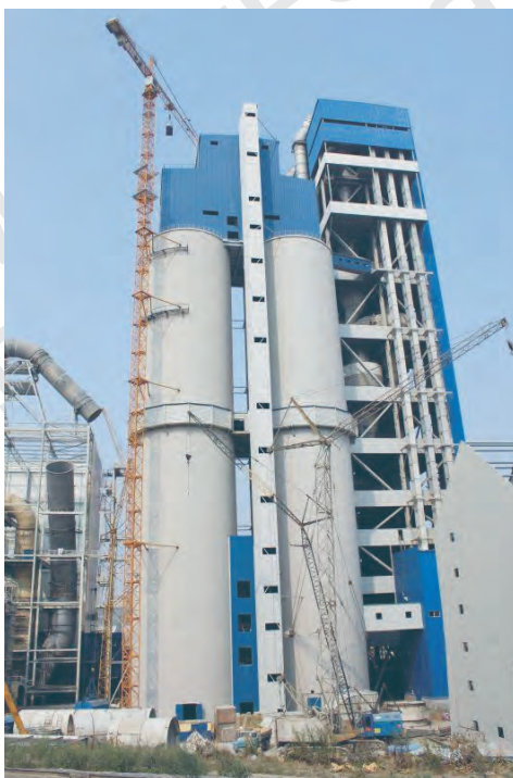
The calculation scheme of silo structures and the constructed “industrial skyscrapers”: 130-meter tall cold end of kiln and 80 m tall silos.
