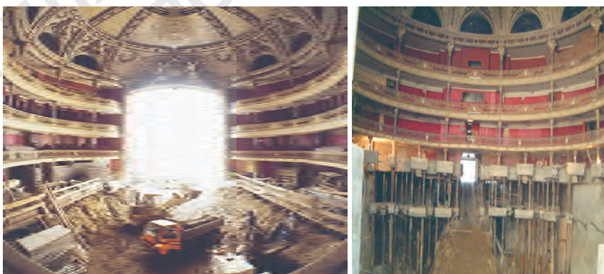
A. Pinto: construction of the second stage under the stalls of Teatro Circo in Lisbon.
