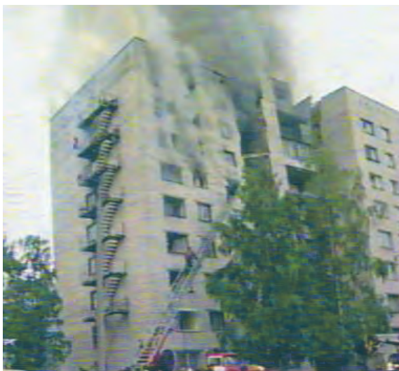
The house on Dvinskaya Street before collapse.
