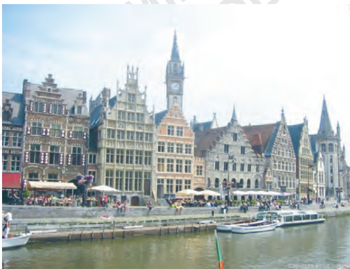
Reconstruction of historic buildings in Ghent (Flanders): the preserved historic facades conceal multilevel underground space and a comfortable hotel with restaurants.
