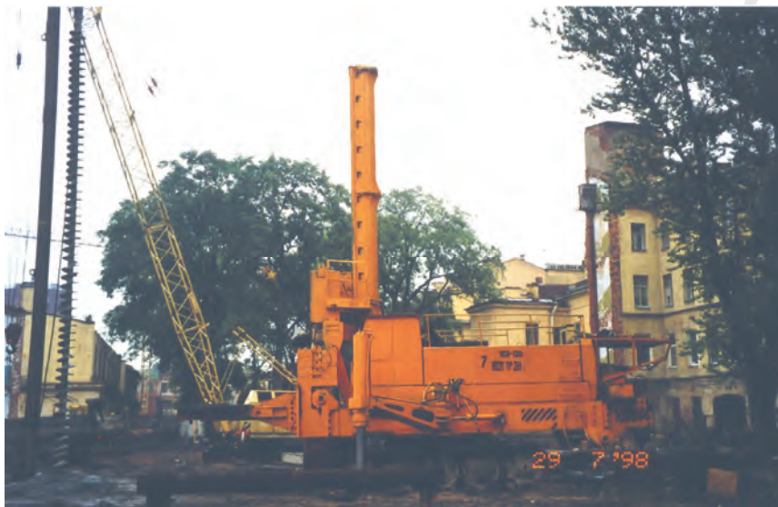
Pile pushing rig YCB120 M.
