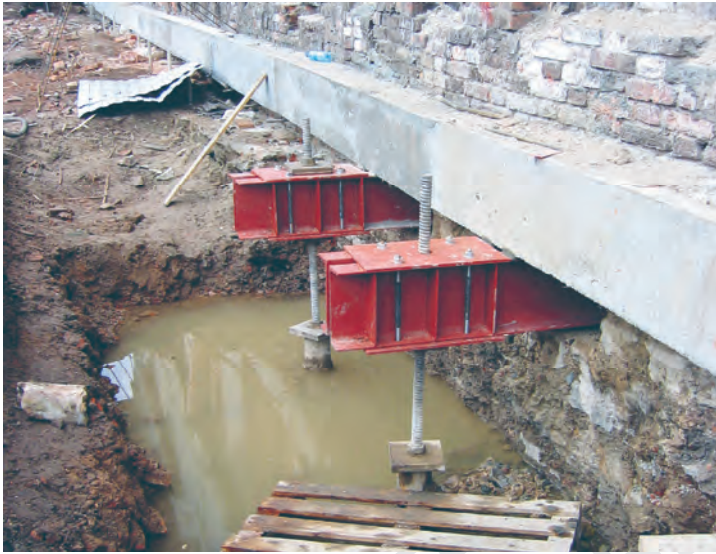
Insertion of beams under the waling and transfer of load to the pile.
