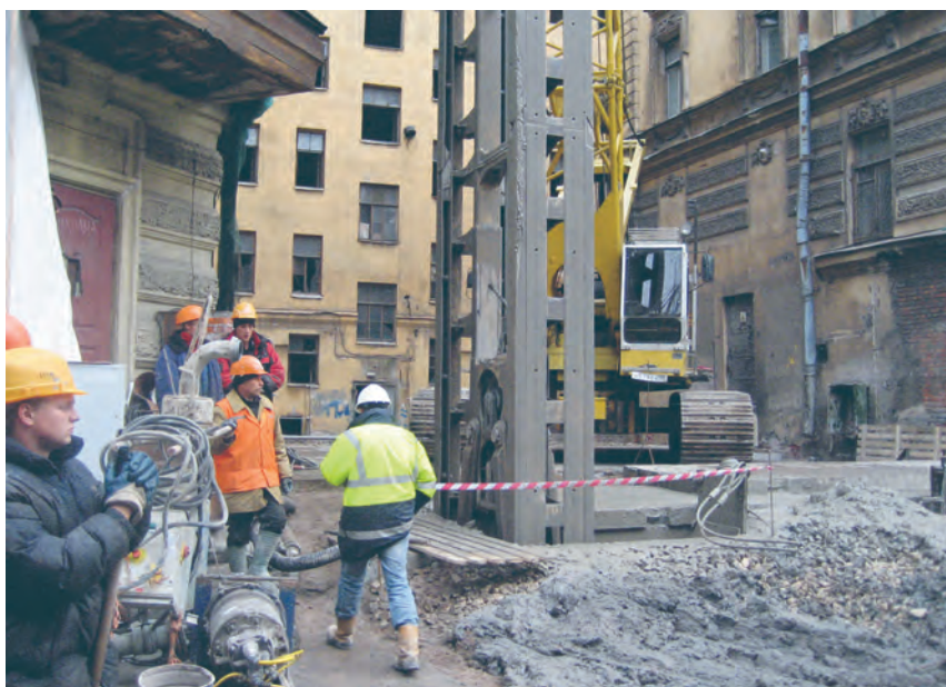
Zoologichesky Lane. First trial of diaphragm wall construction in adjacency to existing buildings (the experiment was carried out on the buildings subject to demolition).
